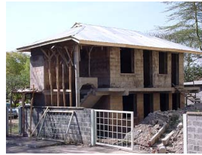
Fig. 2 Double-storey rammed earth building and single story eco-house under construction
