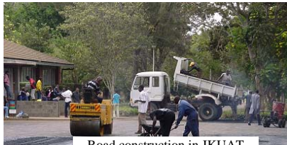
Road construction in JKUAT
